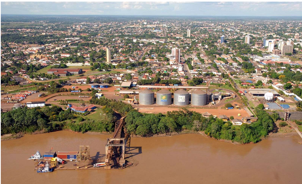
Figure 7: Aerial view of Porto Velho with its fluvial port in front (July 2007)
