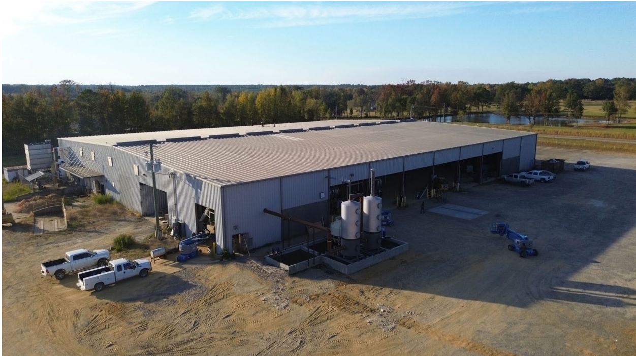
Figure 2- View of BluSky's AR1 50,000 sq/ft plant in Warren, Arkansas
