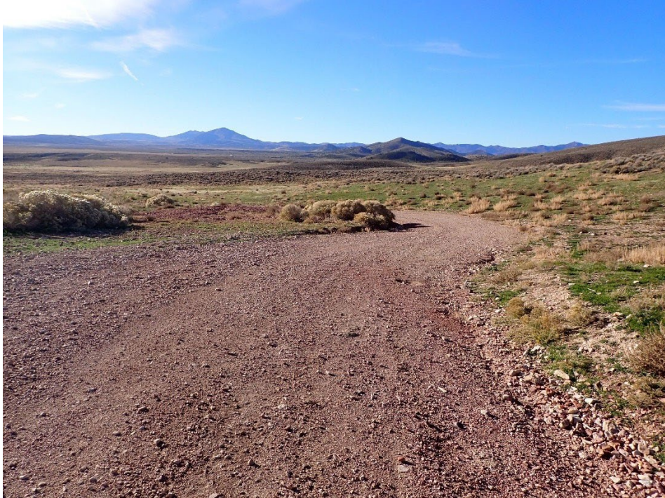
Figure 2: Road conditions within the Property area
