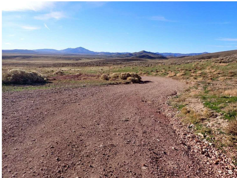
Figure 5.3: Road conditions within Vernon Hills Project area.
