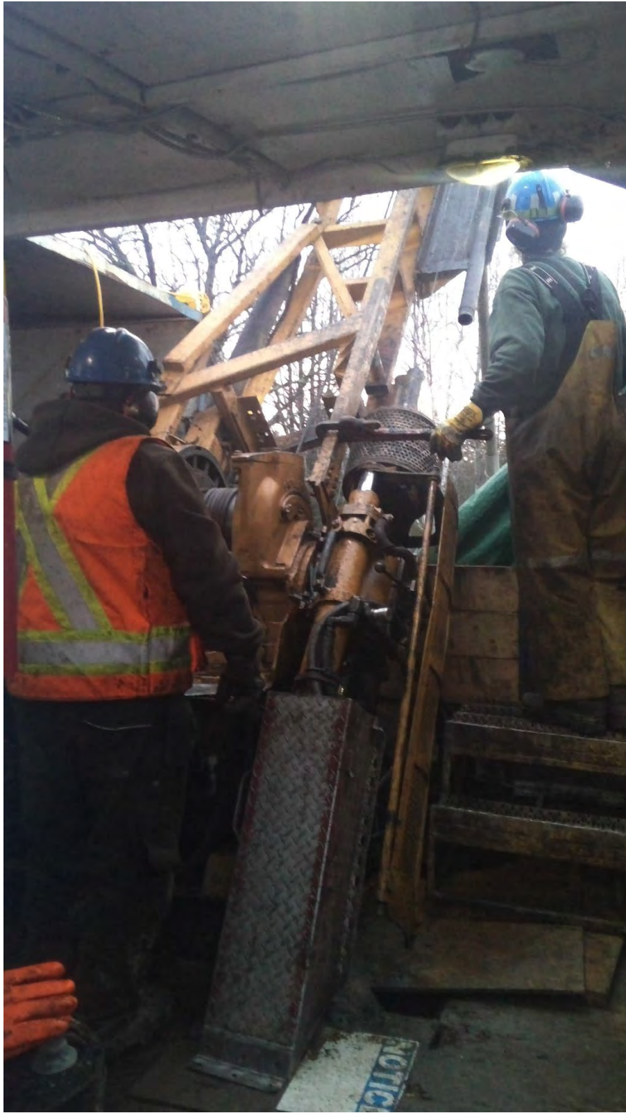
Figure 35 . Pulling core tube
