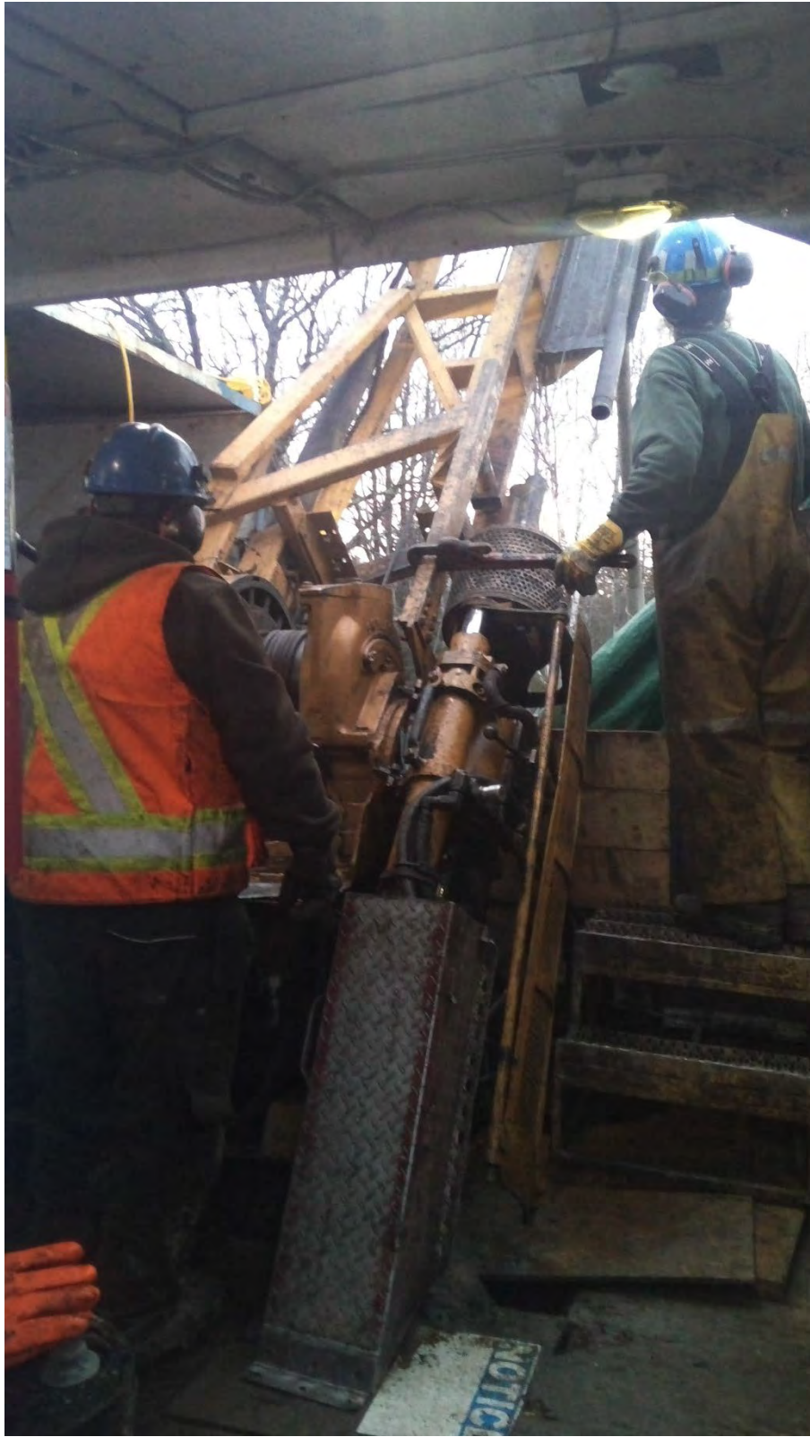
Figure 35 . Pulling core tube
