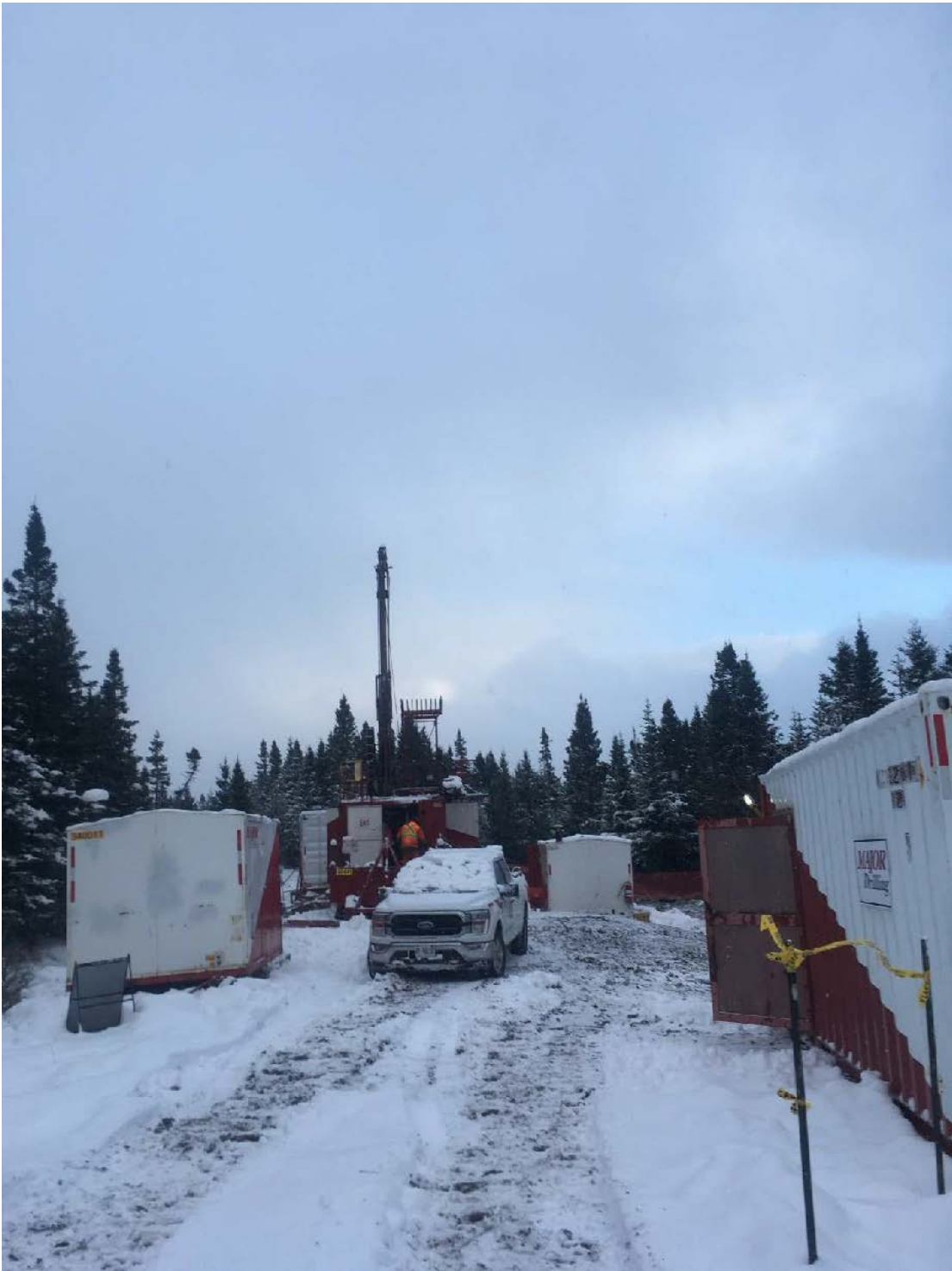
Figure 1: Core Hole 2 Drill Rig
