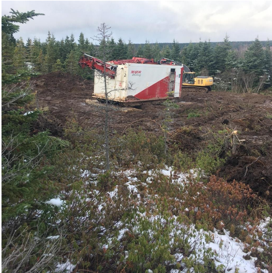
Figure 1: First Pad location with drill rig in place.
