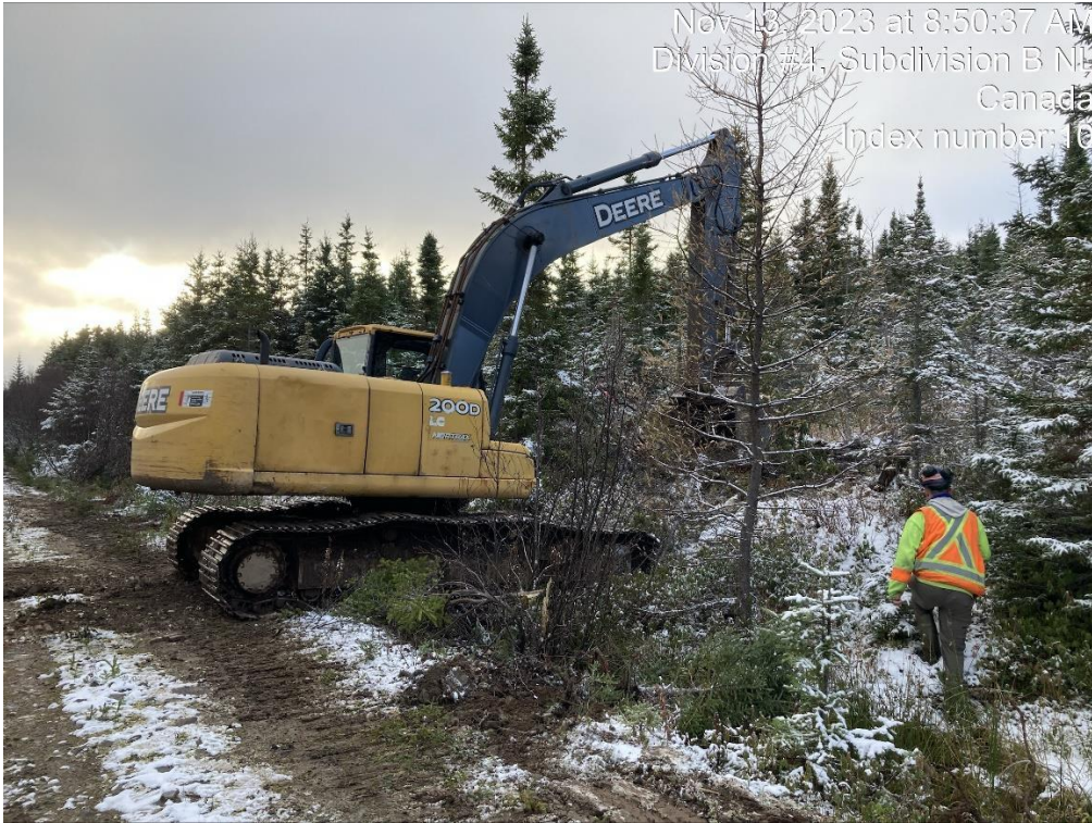
Figure 1: Rig pad being spotted and cleared.
