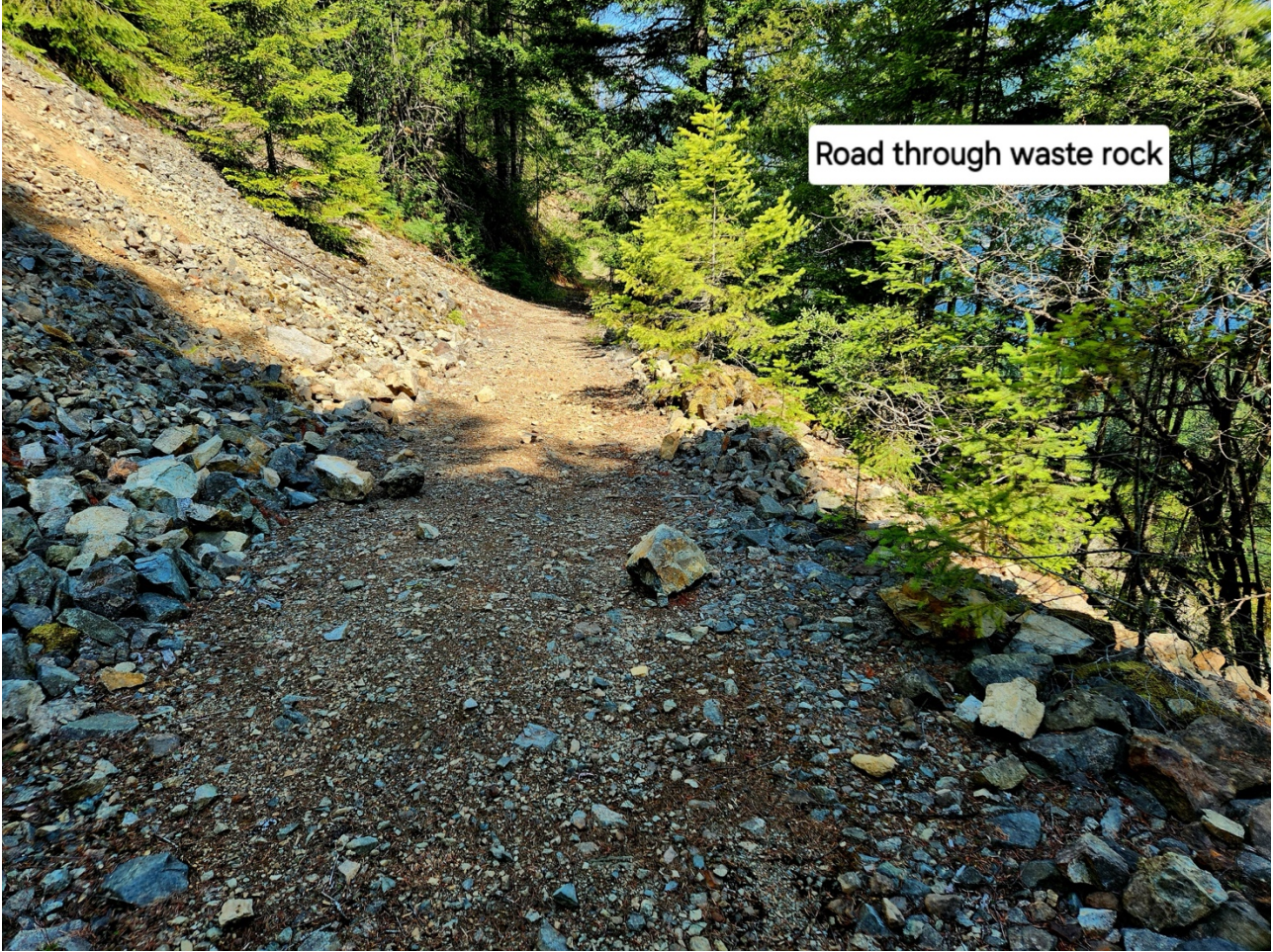
Photograph 2 – access road running through waste-rock
