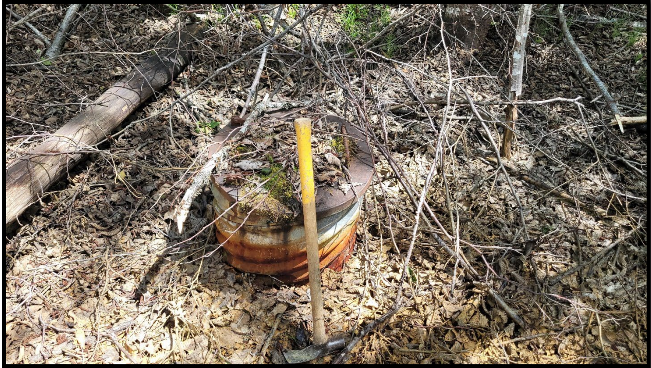
Figure 12-4. Overflow drainage culvert at the lowest elevation of the stored waste and mineralized material from the underground workings (taken June 8, 2024; Station SW24-5, 5414610N, 433603E, NAD 83 Zone 10).
