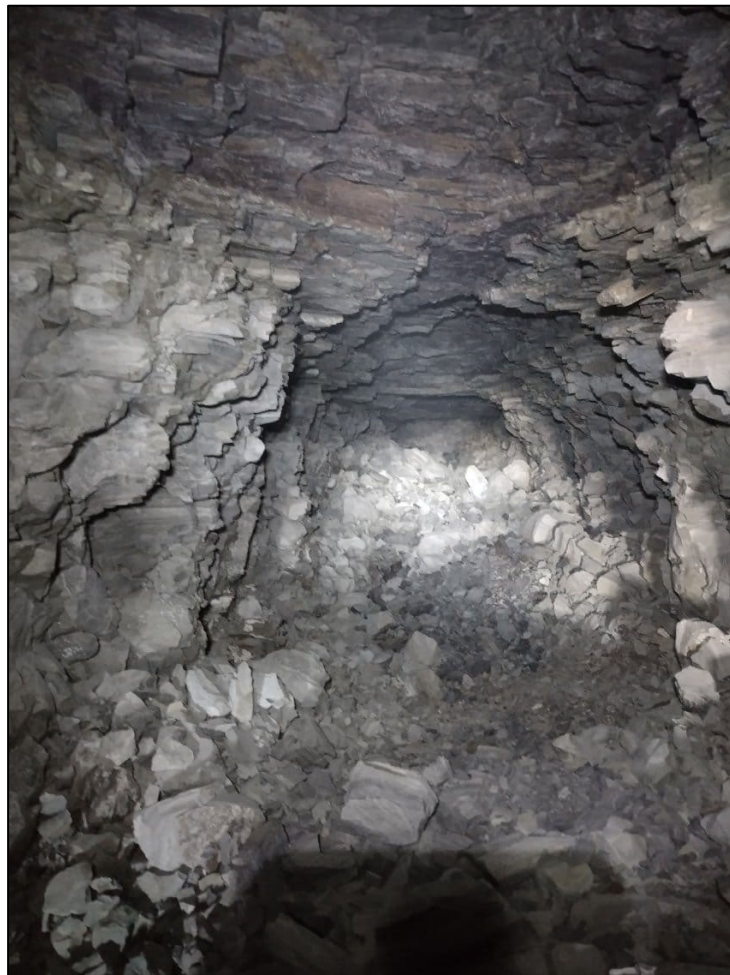
Figure 3 – Inside the Ceciliate workings
