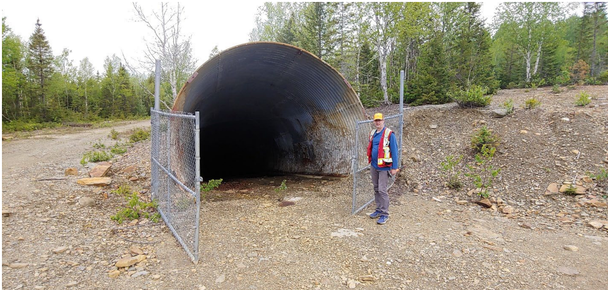
Figure 12.3 Historical portal to underground workings from the June Site visit.
