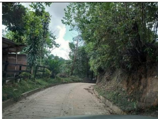
Concrete access road
