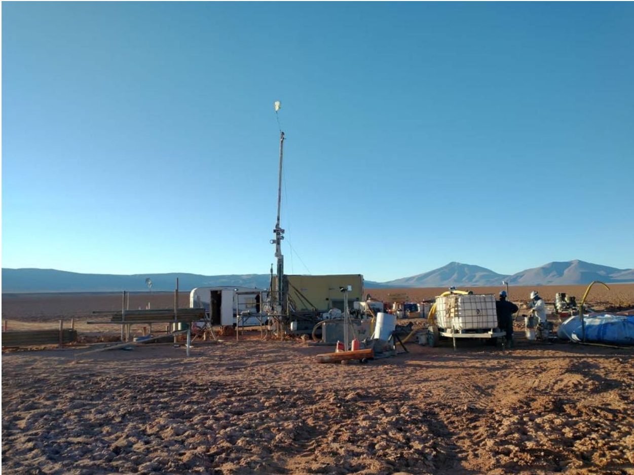
Figure 4. Drilling at Pocitos 1 Lithium Brine Project (Salta, Argentina)
