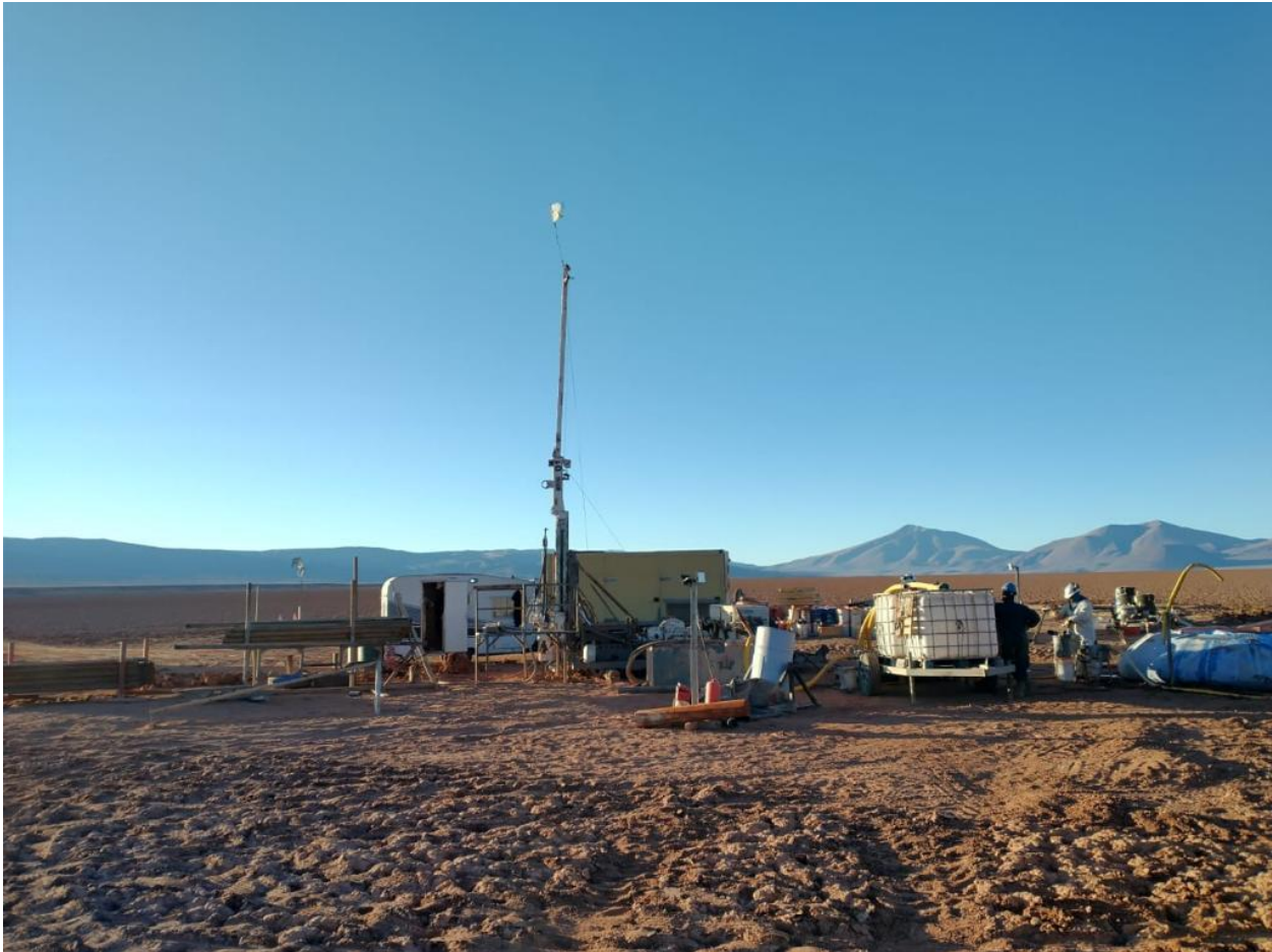
Figure 1. Drilling at Pocitos 1 Lithium Brine Project (Salta, Argentina)
