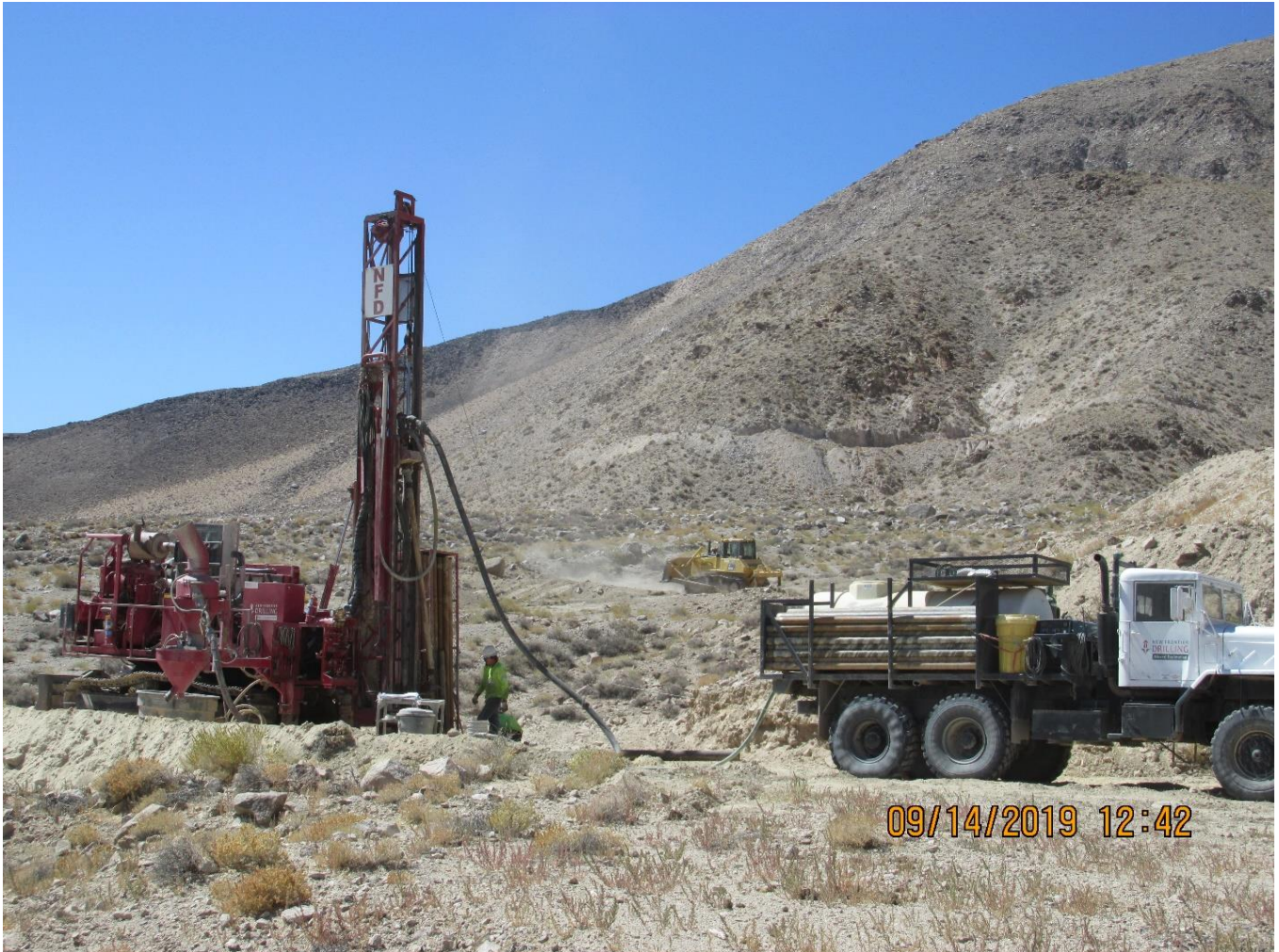
Figure 8 - 2019 Drilling Project Photo provided by Carson River
