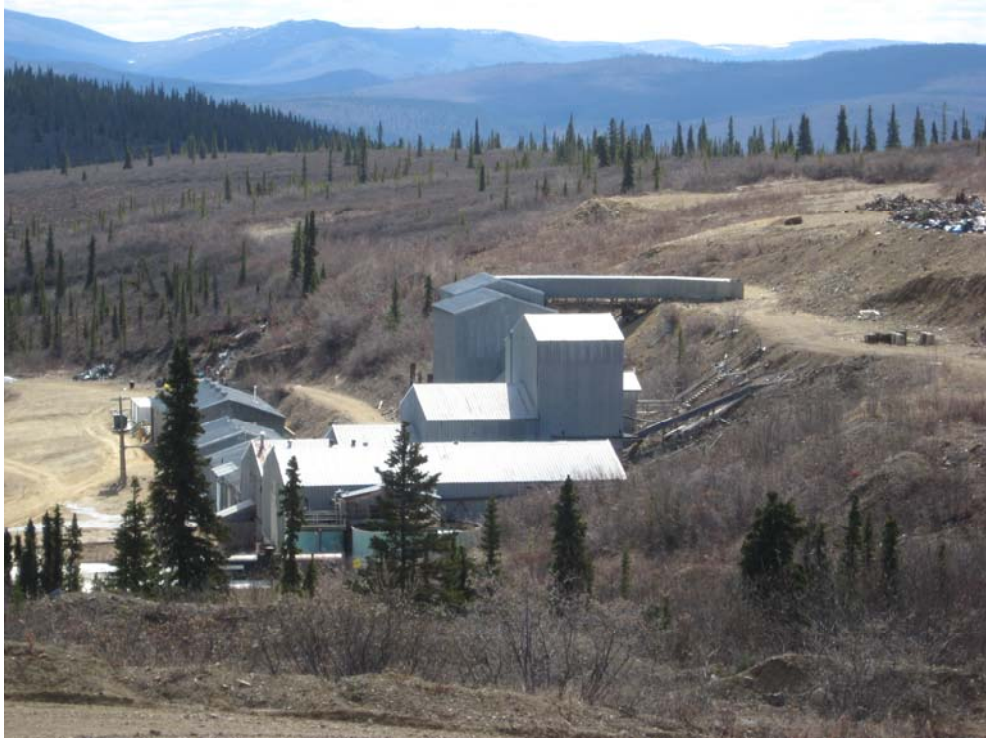
Mt. Nansen Mine. Looking West
