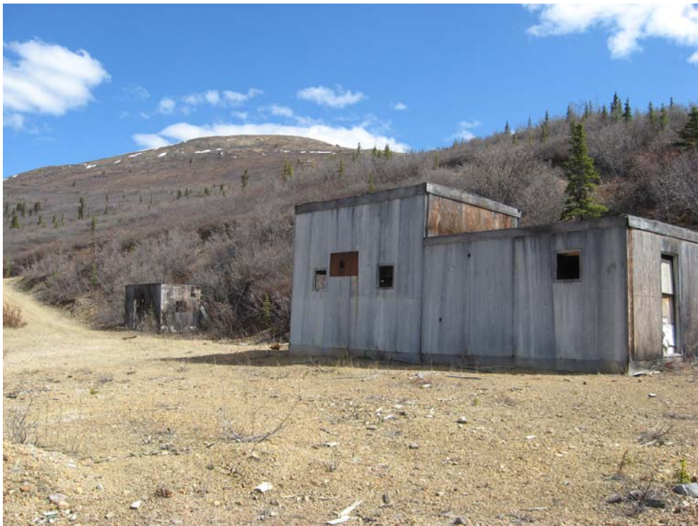
Abandoned compressor building at Upper Webber Portal. Looking East.
