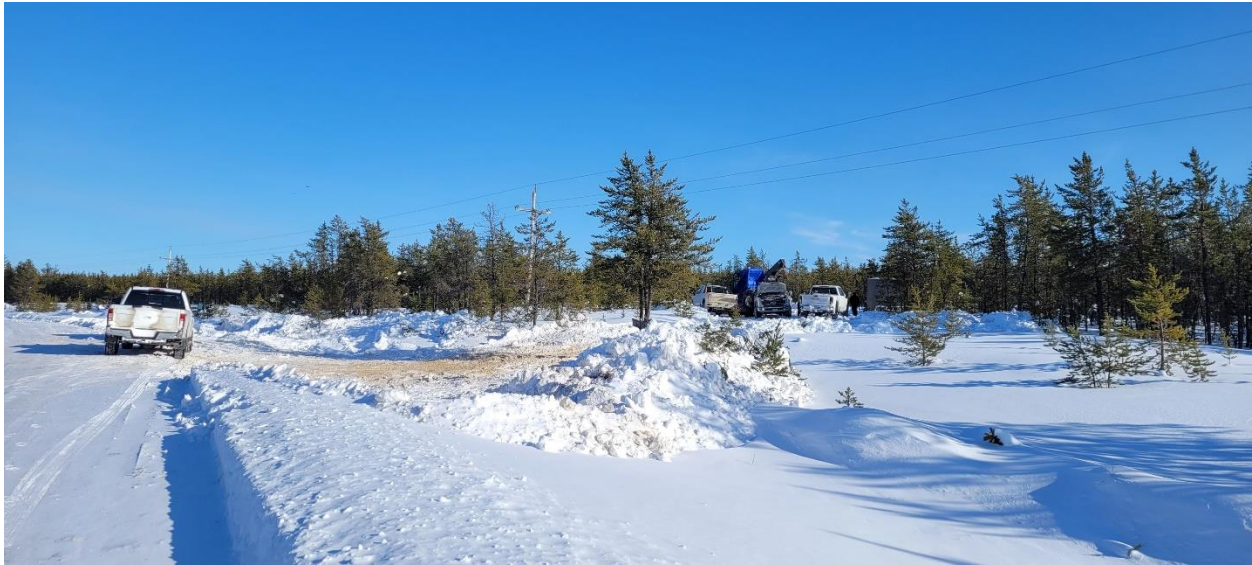
Figure 3. Crew mobilizing equipment to KLS drill site.
