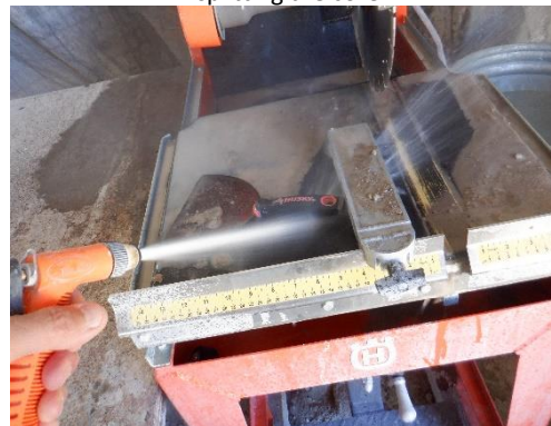
washing the table saw for the next batch for cutting
