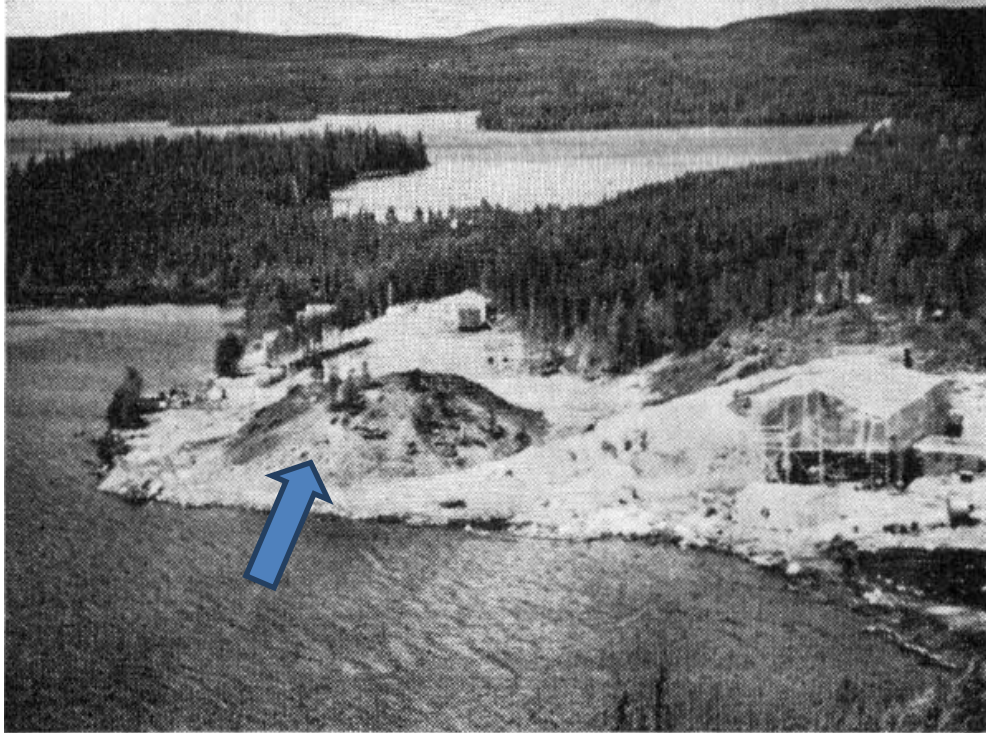
Figure 6-1 The Rottenstone Outcrop and Mill; circa 1965 looking north (pre-mining)
