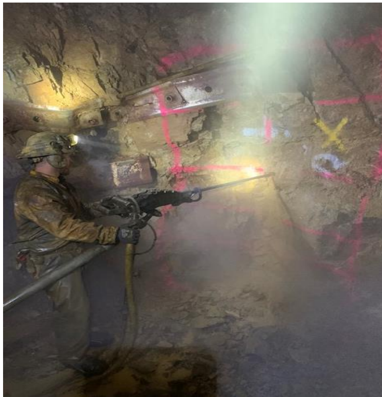
Figure 2: Underground drilling underway to establish new drill bay at Silver Strand
