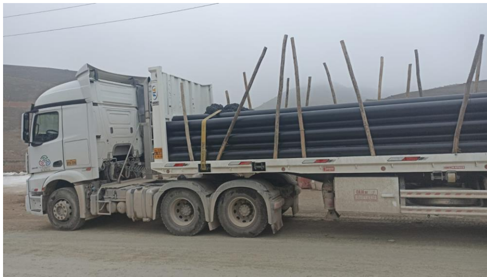
Picture 1. - 3,000 metres of 8-inch piping mobilized from Arequipa to Chachas. October 5, 2023
