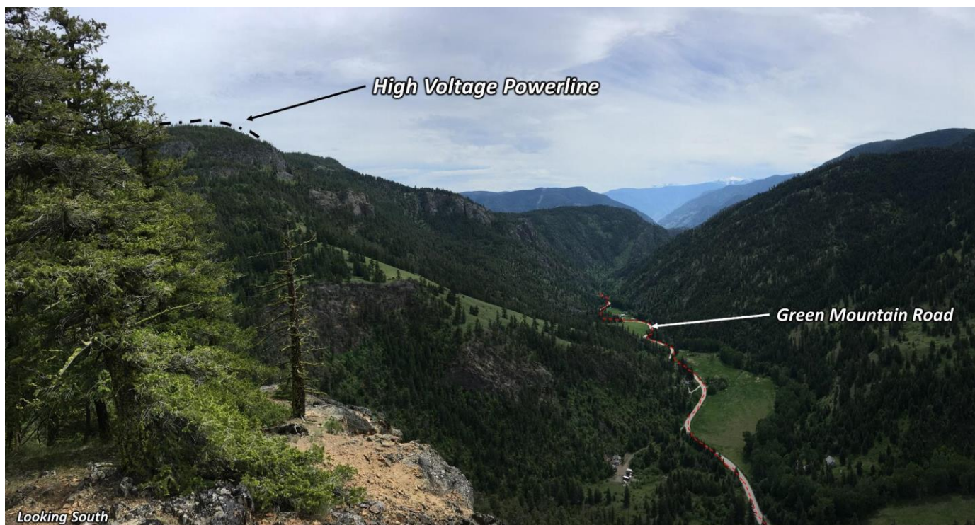
Figure 5.4 High Voltage Powerlines and Green Mountain Road - looking south
