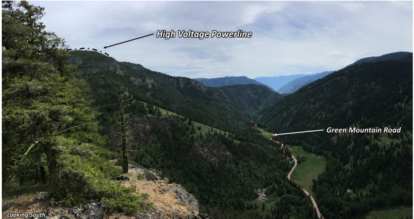
Figure 5.4 High Voltage Powerlines and Green Mountain Road - looking south
