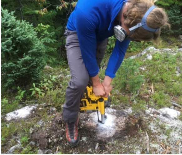
Figure 12-8: Geologist Tom Dyakowski drilling hole HDH-2 in quartzite (UTM 384531E 5294697N, claim 2404904) with the Dewalt hammer drill 20V MAX and dust extractor system D25303DH
