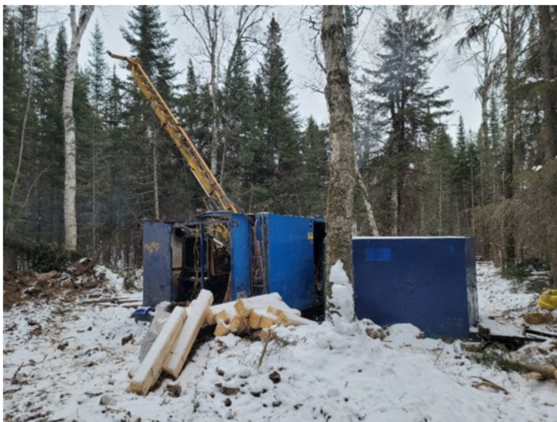
Figure 1: Drill Rig at Echum Project
