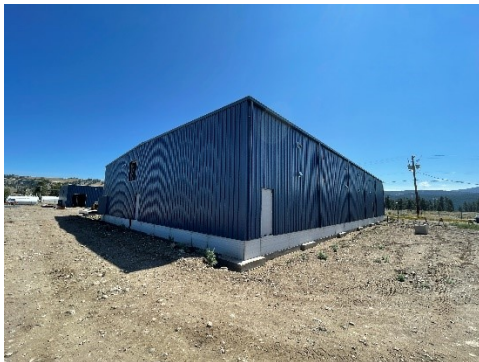
Figure 2 - Building 261 NE view
