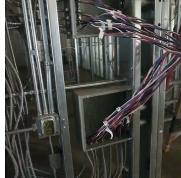
Figure 5 - Electrical Rough In
