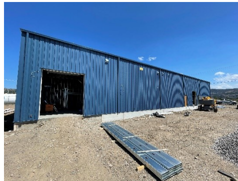
Figure 1 - Building 269 North view
