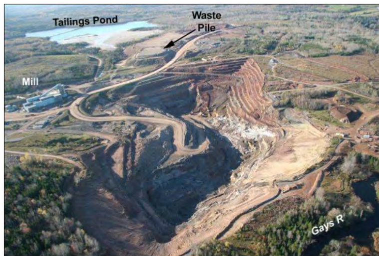
Figure 23-1: Gays River open pit mine and mill (ca. 2012)
