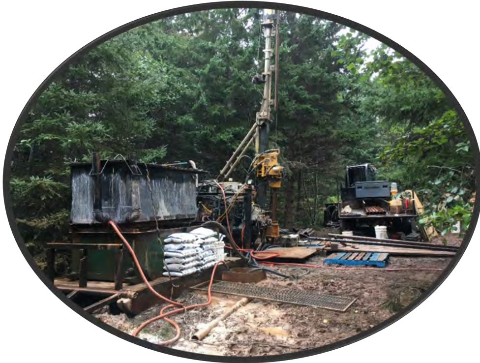
Drill equipment and setup with salt-brining tank at DDH: 18-GHR-005
