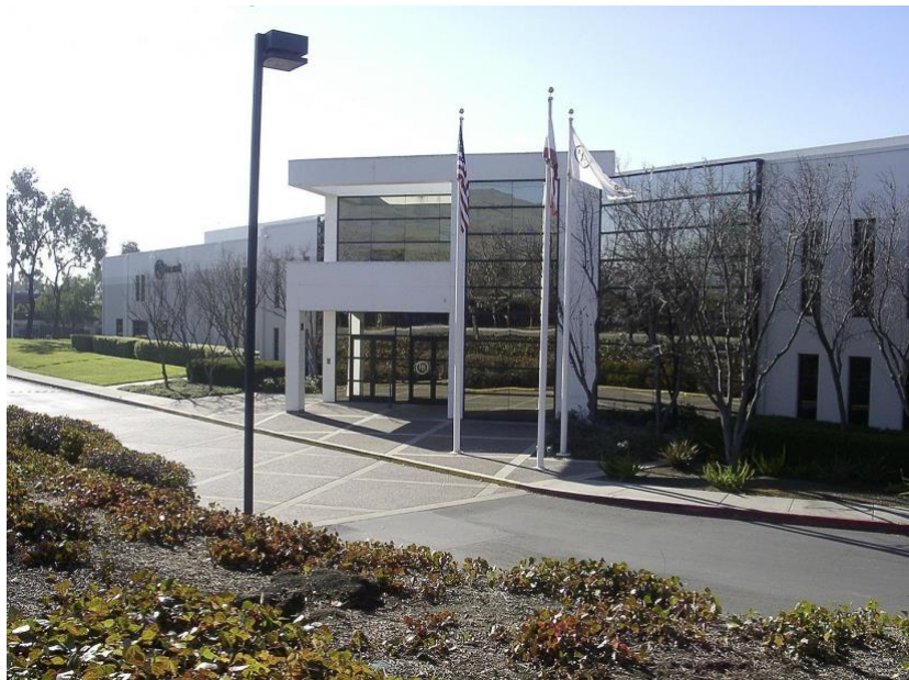
Hurricane Data Center where Impact’s servers are hosted
