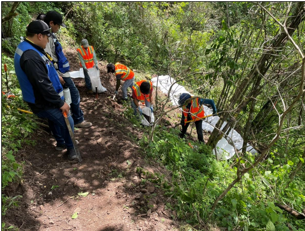
Photo 1. Drill pad preparation at Palos Verdes
