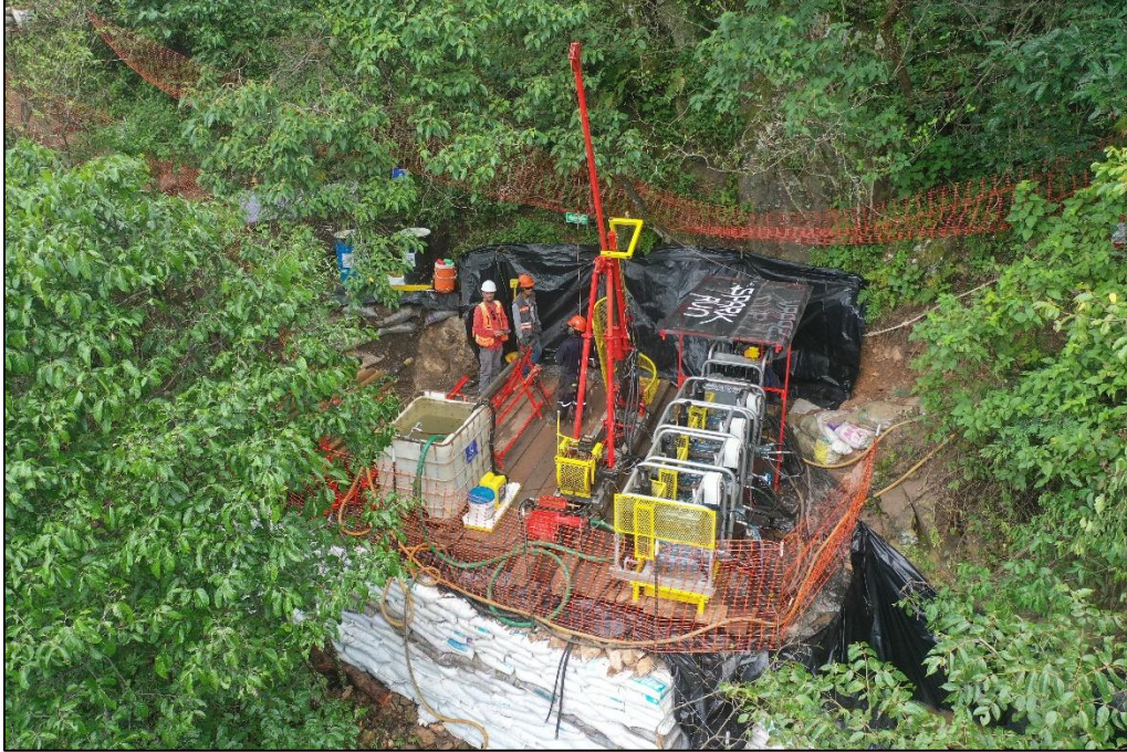
Photo 2. Drill installed on drill pad at Palos Verdes
