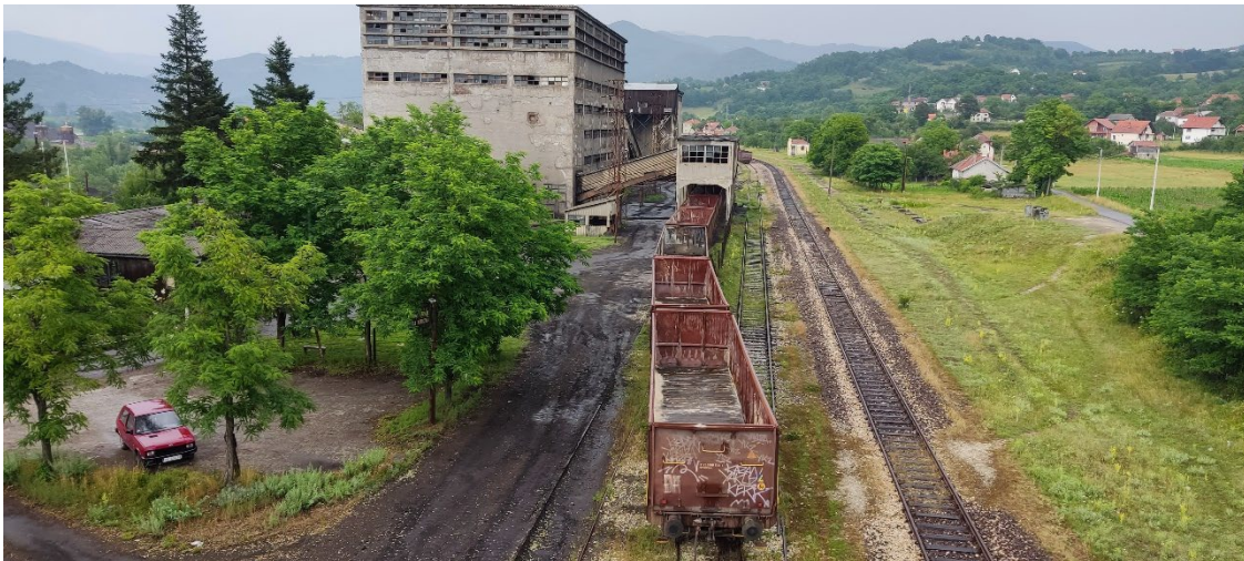
Figure 18-5: (For location, see Figure 18-1 label “P4”) Existing Industrial Land adjacent to mainline railway and sidings to be refurbished and utilized for load-out. Photo looking towards the north-northeast. June, 2022.
