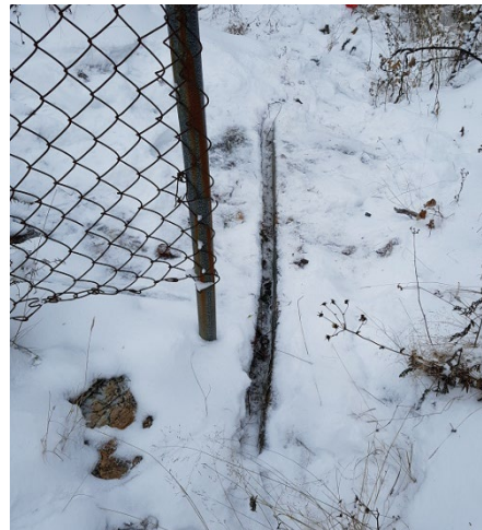
Photo 5: Trench at Sample KG19-04
