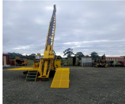
CS 1000 drill rig in Tasmania with mast up
