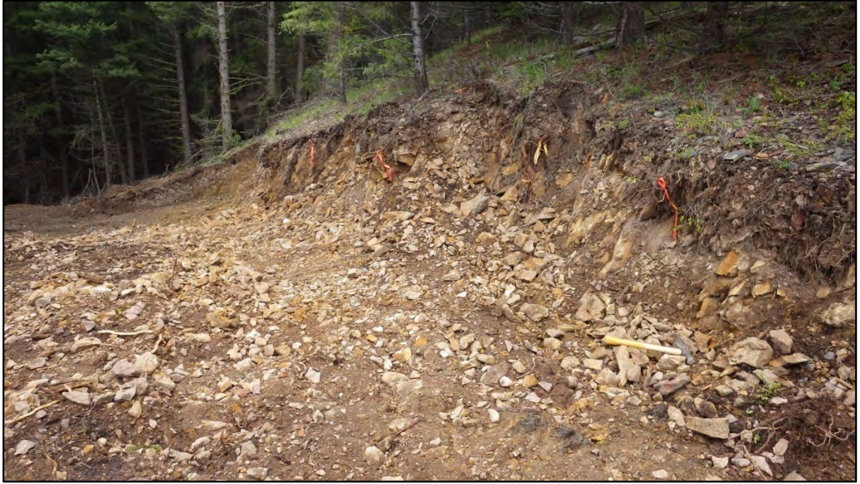
Figure 24: D Area (site of recent trenching)
