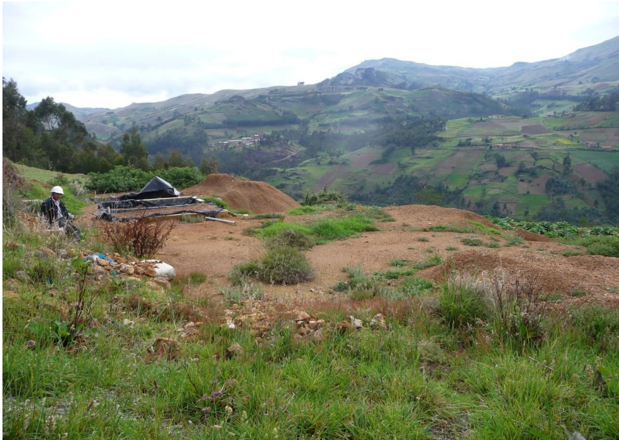
Figure 8.3: Areas excavated along strike of MZ4 structure
