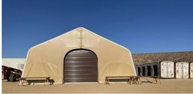
Figure 8-4: Core Shed and Quick Log Station
