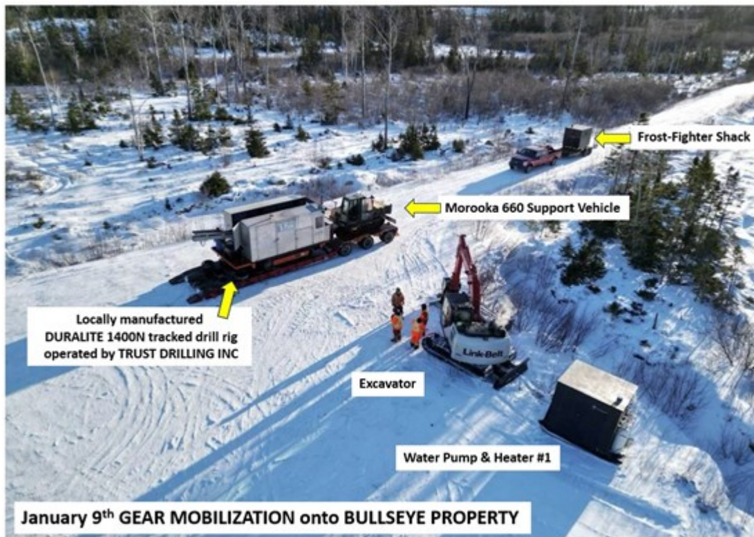
Photo 1: Gear mobilizing onto the Bullseye property.
