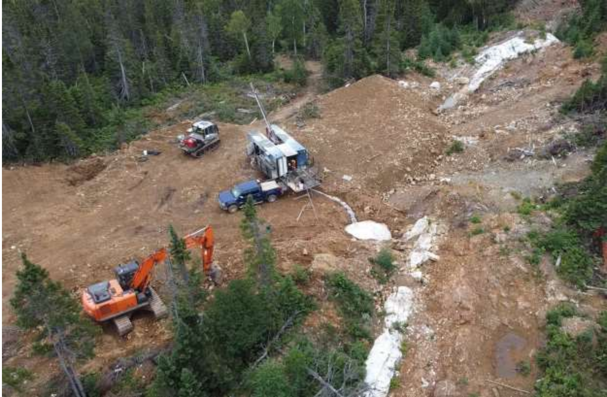
Figure 1: Drill set up at Jonathan's Pond
