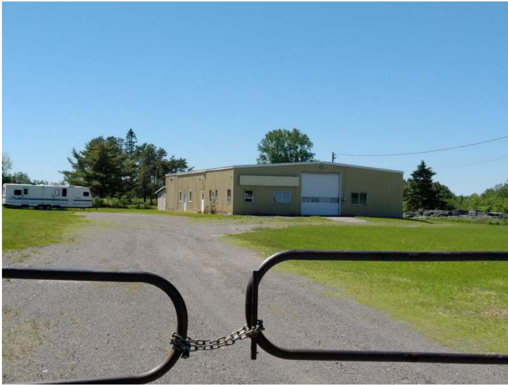
Figure 12-19 Northstar's secure drill core logging and storage facility.
