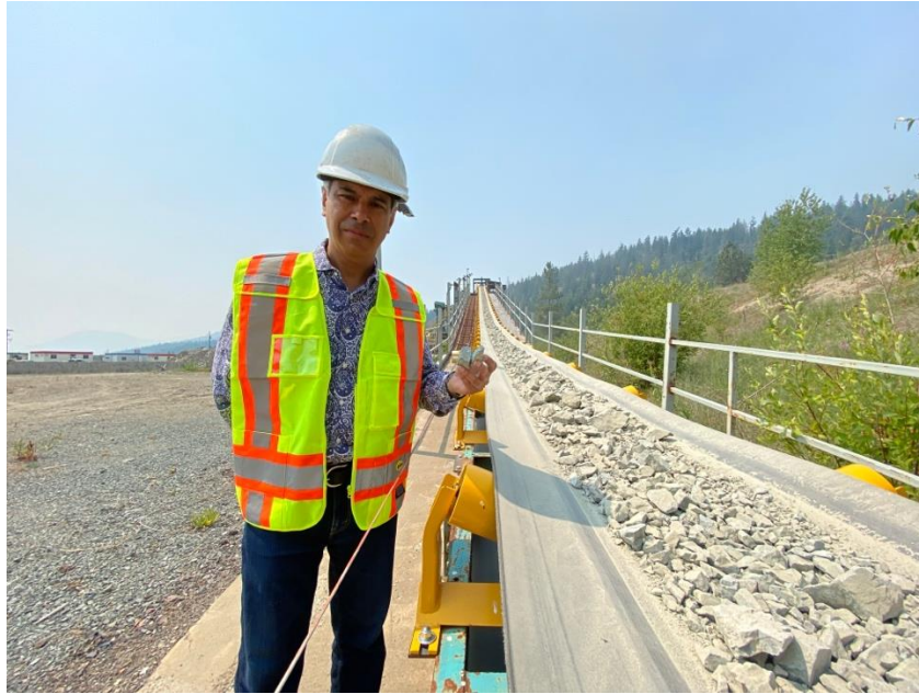
Blue Lagoon Resources President & CEO, Rana Vig, standing next to conveyer transporting Dome Mountain mineralized material from Nicola's primary crusher to its secondary crusher
