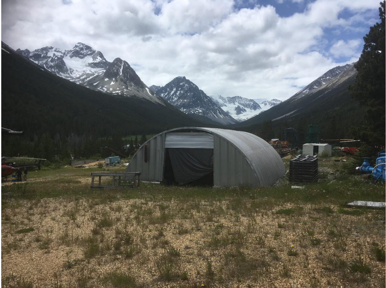
Figure 18-5: Maintenance Quonset Hut
