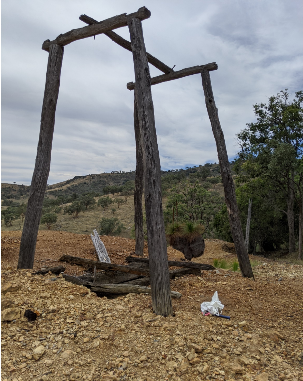
Figure 9.1 Old Wooden Headframe at abandoned Torny Mine Shaft
