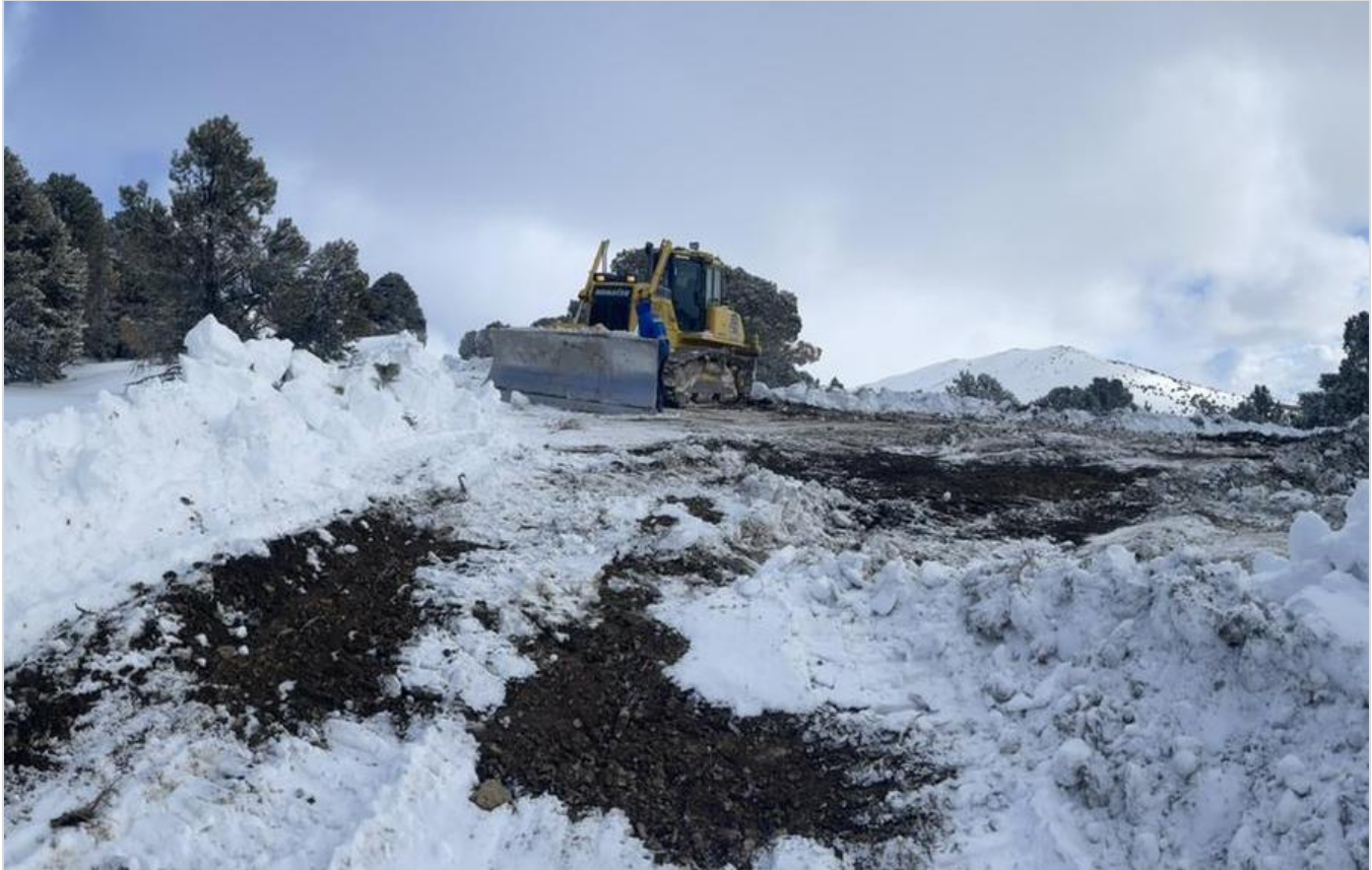
Figure 1: Clearing Pad for Planned Drill Hole T2301
