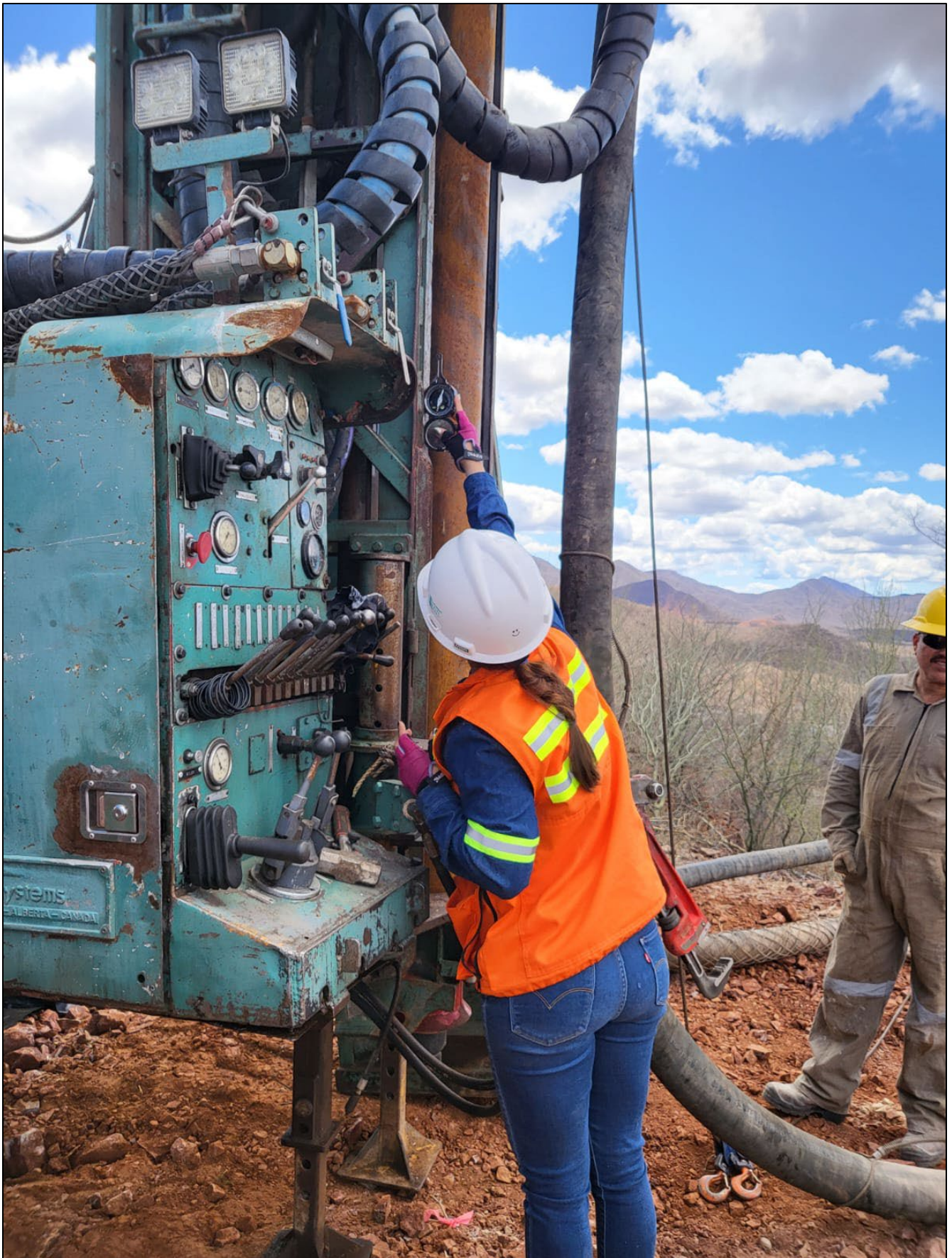
Photo 2. Lining up drill hole JES-24-73.
