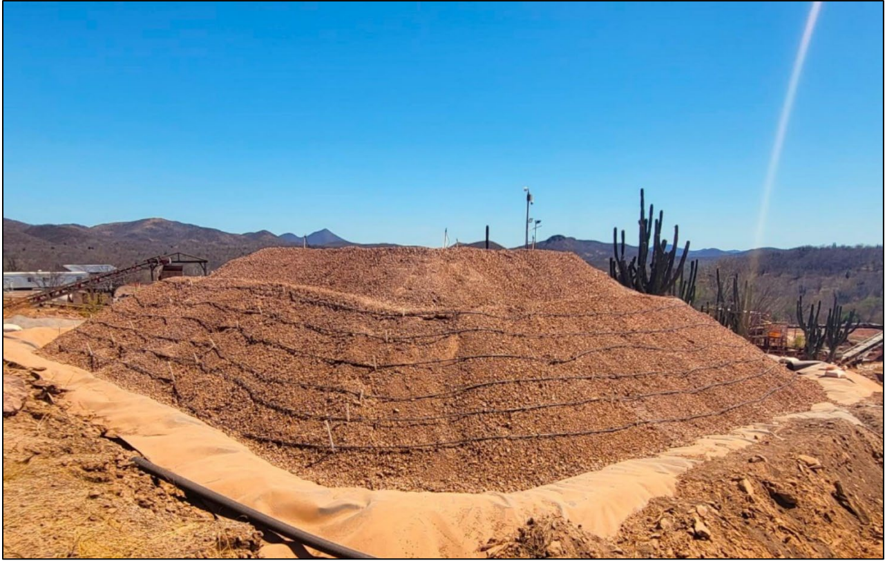
Photo 1 & 2. Bulk Sample heap leach pile during irrigation setup.
