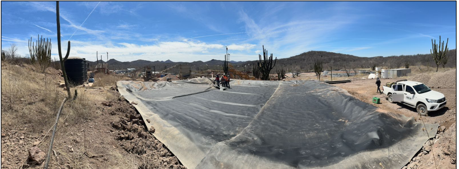
Photo 1. Leach Pad Liner set into place prior to stacking of material.
