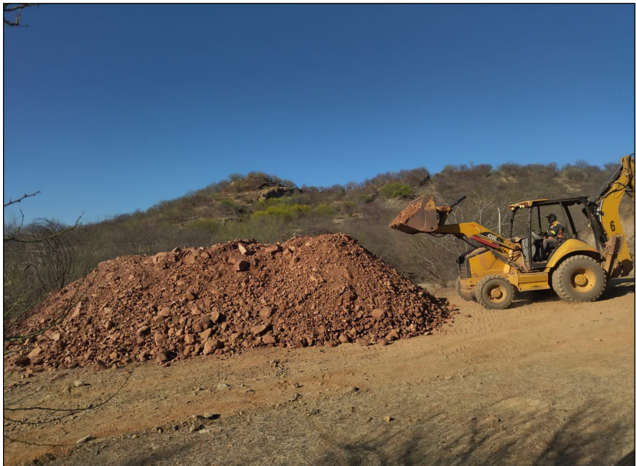
Photos 1 & 2. Above, Trenching for Bulk Sample at 4-T, channel sampling averaged 2.2 g/t Au and 31 g/t Ag over the 25-meter trend. Below, a stockpile of bulk sample material – Main Zone.
