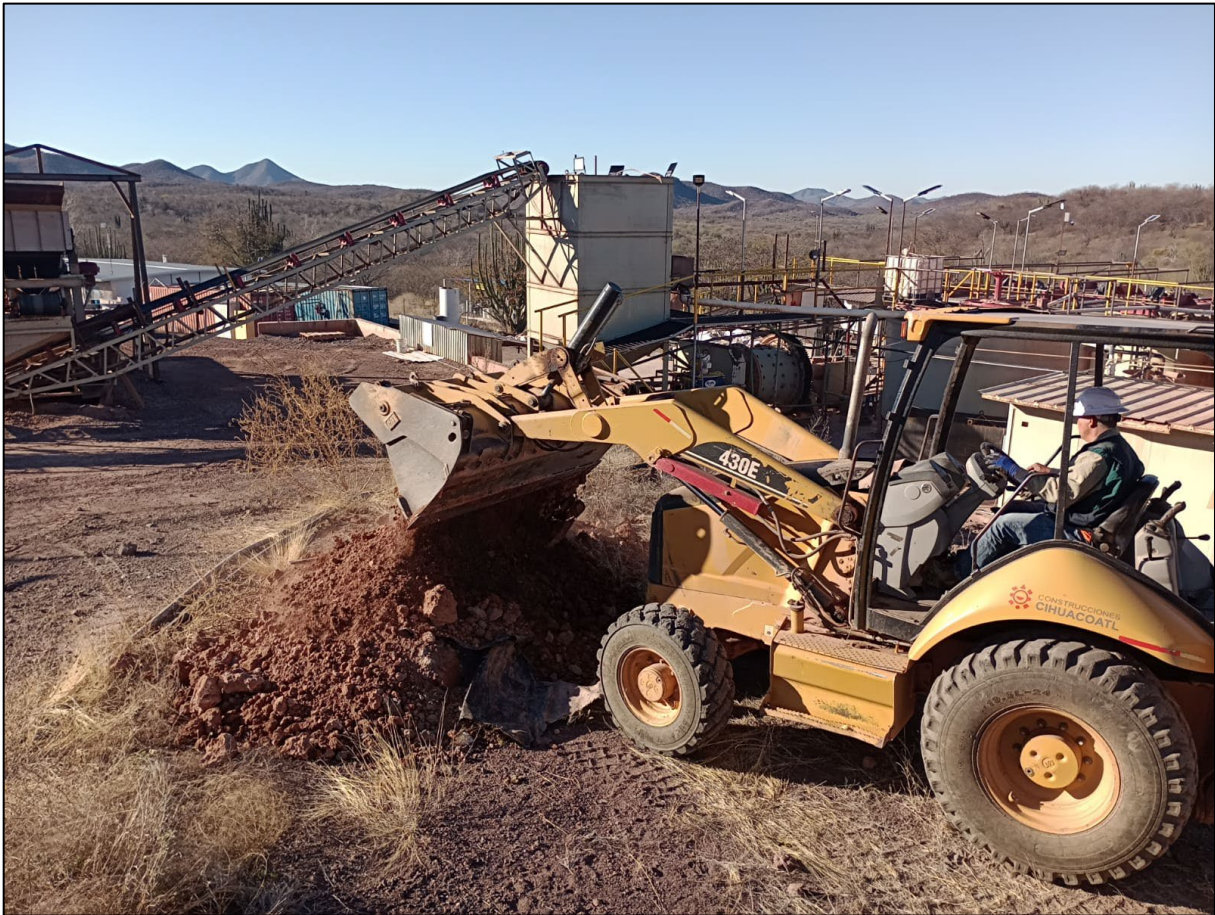
Photos 1 & 2. Above, Ground conditioning for heap leach pad. Below, Absorption Tanks for treating solution.
