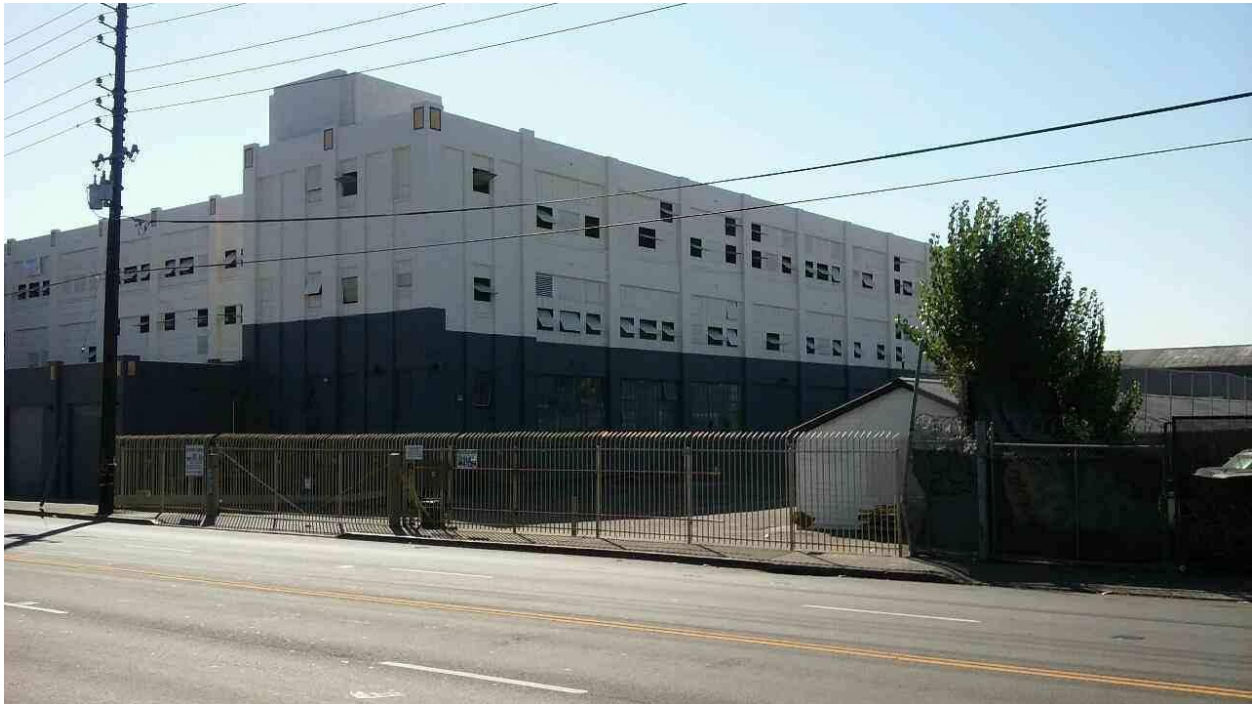
The northwest corner of The Oakland Tinnery located in Oakland’s Green Zone. Source: Green Sage
